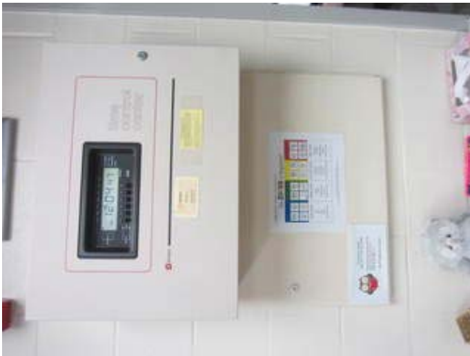
Centralized Clock System
