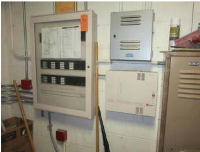
Fire Alarm System Control Panel
