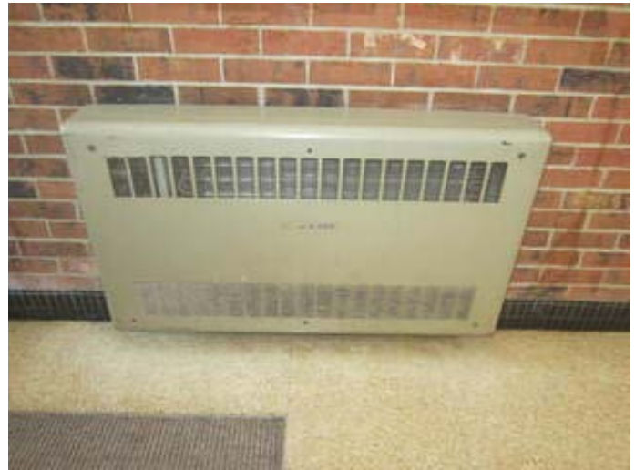
Heating Water Cabinet Heater
