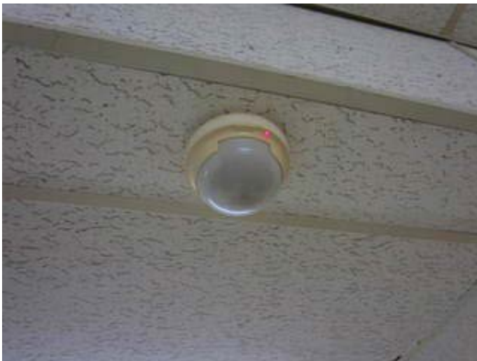
Security System Motion Sensor
