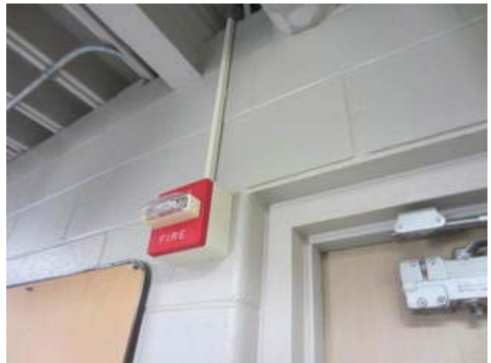
Fire Alarm System Audible Horn Strobe Indicating Device
