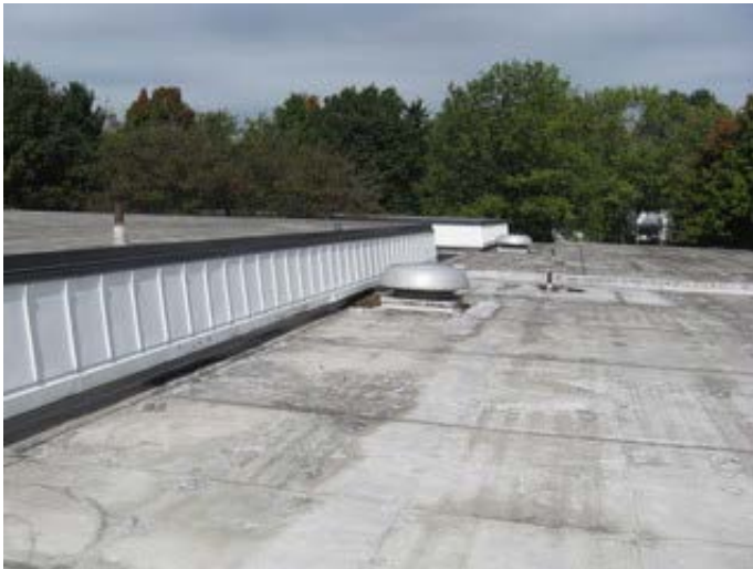
Membrane Roof and Standing Seam Metal
