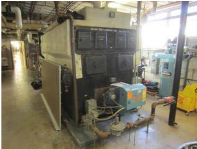
Natural Gas Fired Heated Water Boiler Type System
