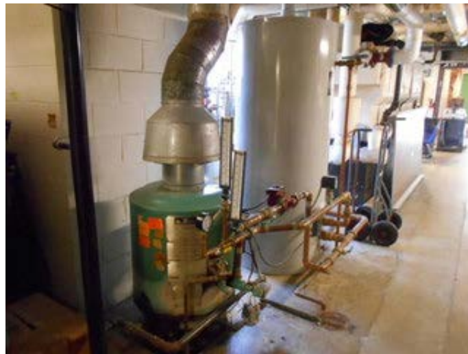
Water Heater with Storage Tank 1968 Original Construction
