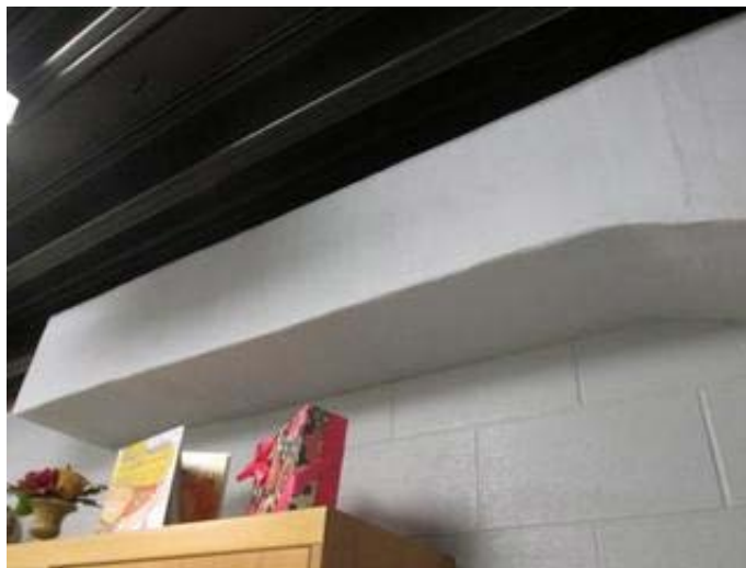
Duct Insulation
