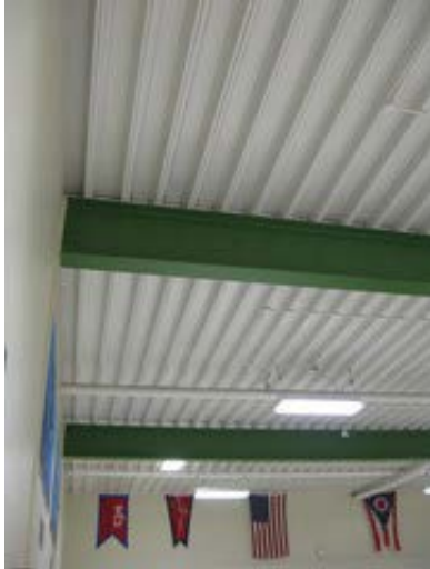
Preformed Composite Structural Metal Deck
