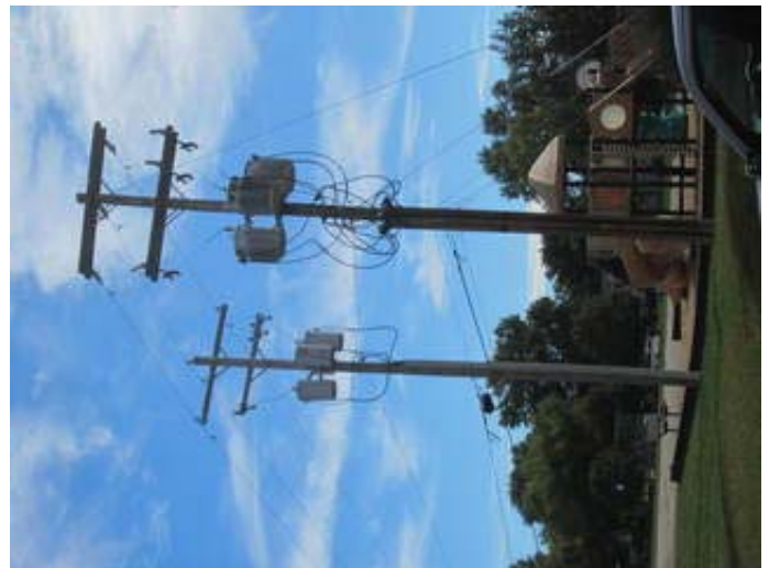
Pole Mounted Transformers
