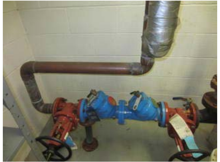
Incoming Domestic Water Service Backflow Preventers
